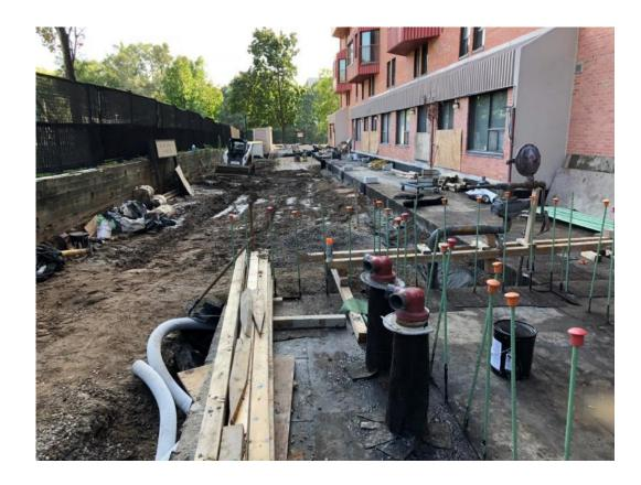
Concrete repairs, install dowels, sandblast, install waterproofing
