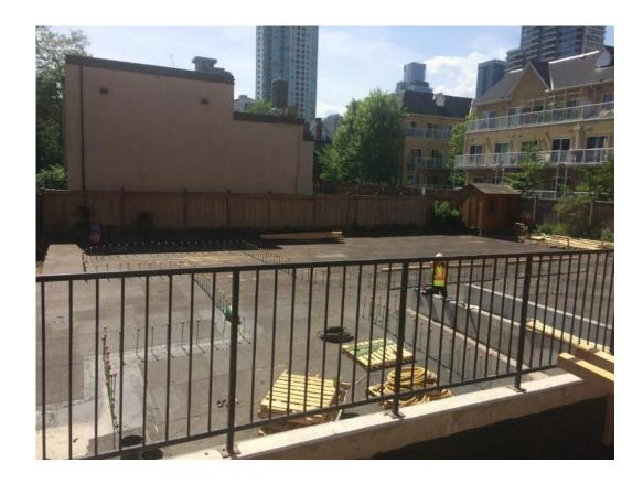
Concrete repairs, install dowels, sandblast, install waterproofing
